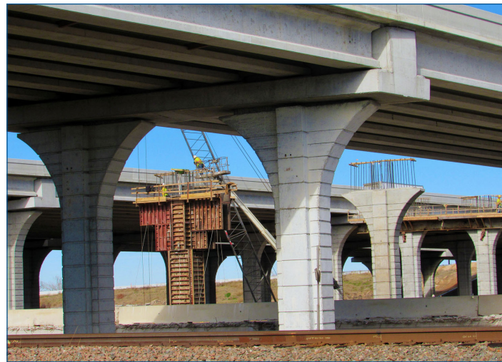
I-69 expansion nears completion in Rosenberg, Texas
